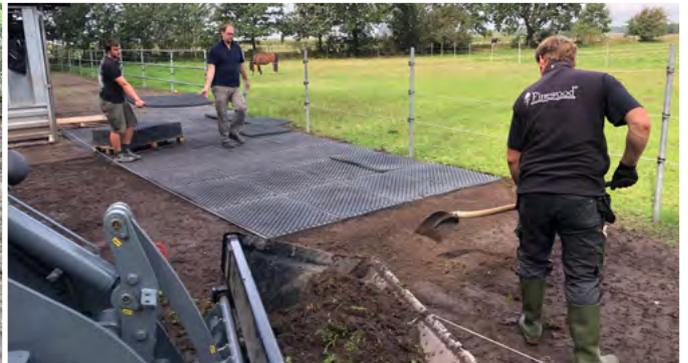
3. Lay the mats in a masonry configuration with a 1 - 2 cm gap between each mat. Cut the mats with a manual or powered saw.
