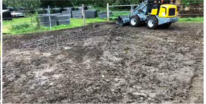
2. Break up approx 5cm of the surface with a strong rake or similar tool. This allows the mat to imprint and fit into the ground.
