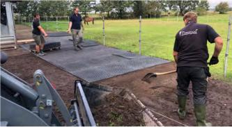
3. Lay the mats in a masonry configuration with a 1 - 2 cm gap between each mat. Cut the mats with a manual or powered saw.
