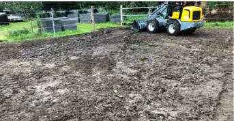
2. Break up approx 5cm of the surface with a strong rake or similar tool. This allows the mat to imprint and fit into the ground.
